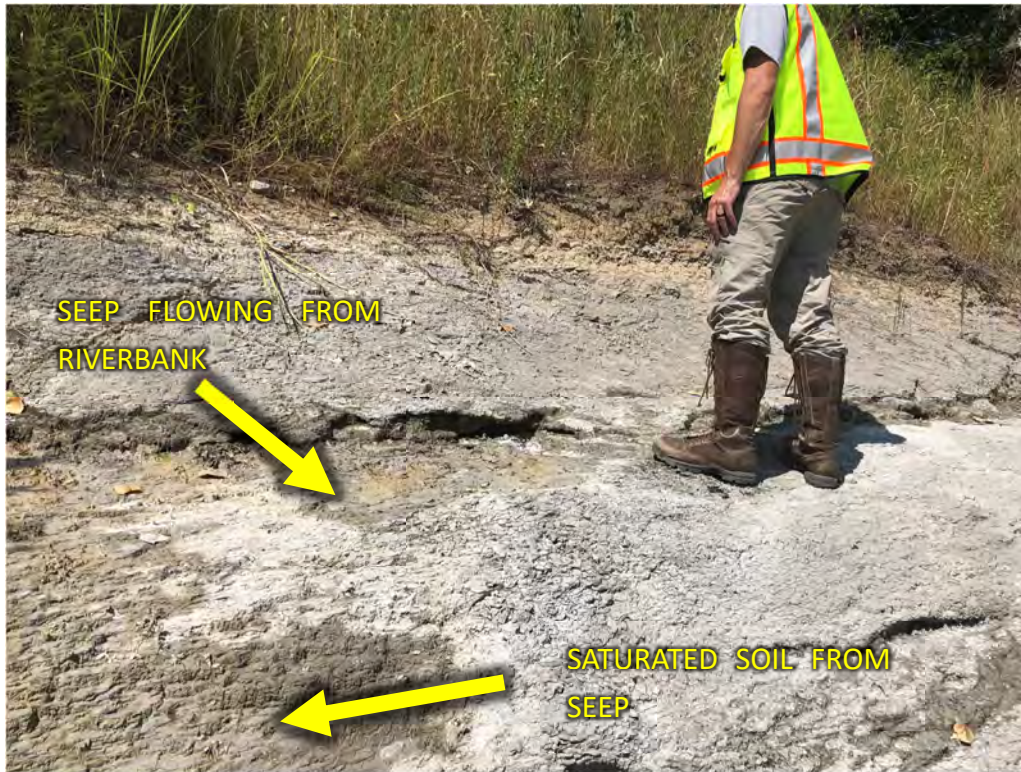
Figure 11. Example photo of seep in existing MC NSR. Note the saturated soils.
